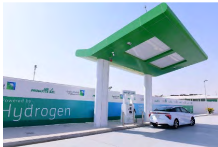
Hydrogen Fuel Cell
