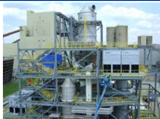
AEP Mountaineer USA - 58 MWth Chilled Ammonia - Coal
