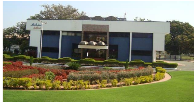
VADODARA MANUFACTURING SITE
